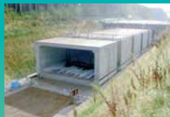
Tunnel Construction under the Stone Circle
