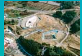
Ongoing Construction of Baseball Stadium
